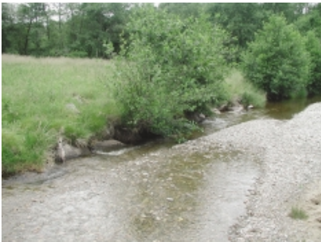
I6a Reinforced bank – toe only; reinforcement is with large boulders (rip-rap). See also E1Ja,b, E1Ka, E1Oa.
