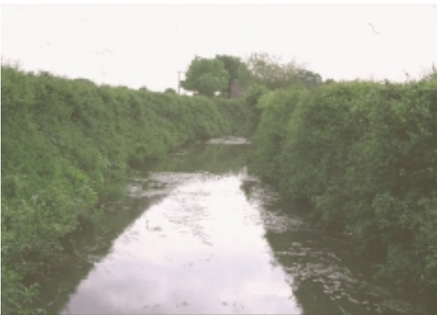
D8a Over-deepened channel – very obvious tell-tale signs are the uniformly sloping, artificially steep, banks and a channel width/bank depth ratio <4:1 . See also E2Aa.
