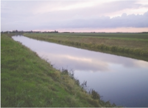
A1a Artificial channel cut through flat fens; site is not part of a river. Note no obvious valley sides.
