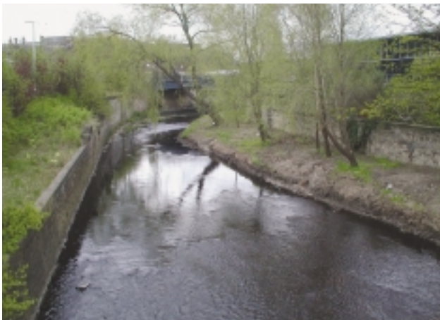
I6c Reinforced bank – record as ‘top only’ on right, and ‘whole’ on left. See also A1c, E1La,b, E1Mb,c (all whole banks).
