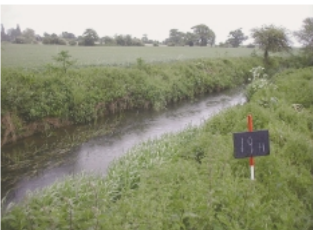
D8c Over-deepened channel – less obviously over-deepened, but with artificially steep, undercutting, banks and the channel width/bank depth ratio is <4:1 .
