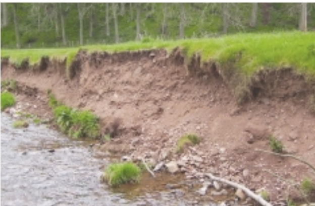
E1Eb Earth bank material; a 'jab' with the ranging pole will not leave a smooth, well-defined, hole.
