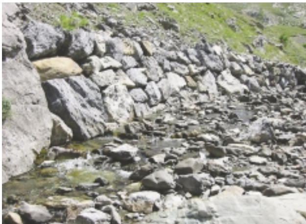
E1Ma Rip-rap bank material; placed (but not cemented), non-regular, blocks. Bank vegetation structure is recorded as bare.
