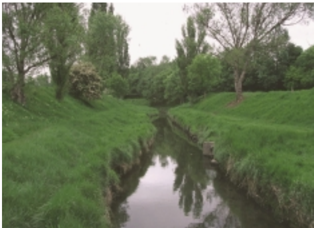
E2Ca Artificial Berm – formed by excavating bank material (here on both sides) to form a two-stage channel. Both the flat base of the berm, and the face of the top of the bank, constitute 'bankface'. See also E1Hb, F18b.
