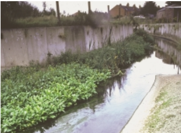
E1Hb Concrete bank material. This example illustrates an artificial berm as habitat creation as part of a flood defence scheme, and this should be noted in Section P.
