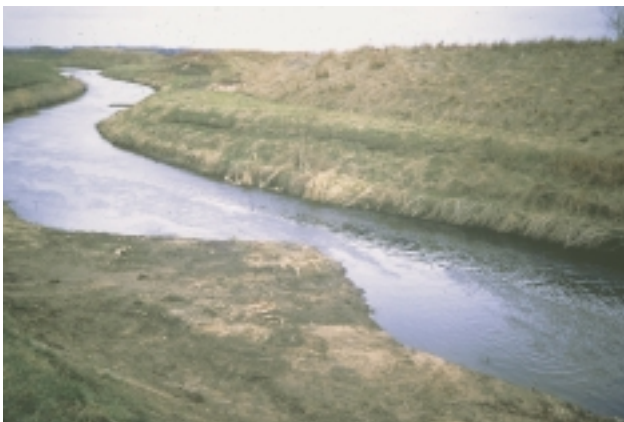
D6a Major deflector/groyne/croy – extends across >20% of the channel width. This example is composed of mixed materials, including compacted earth.
