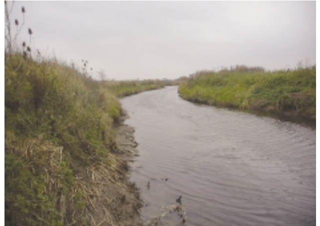
E6b Resectioned channel – typical signs include trapezoidal 45 degree banks and no trees.
