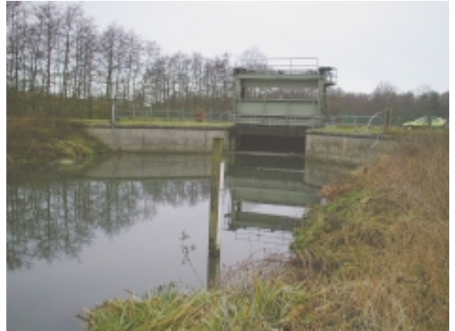
D1b Major weir/sluice – sluice; settings can be changed to influence water levels upstream. Water is impounded upstream.
