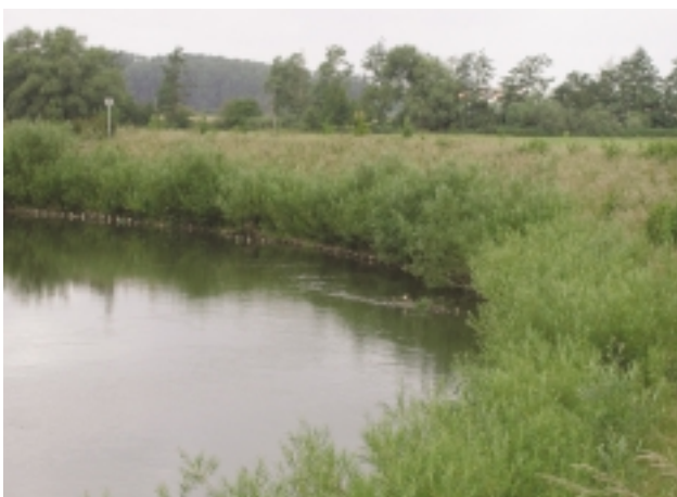
E1Pd Bio-engineering bank materials – live willow stakes. Bank vegetation structure is 'simple'.
