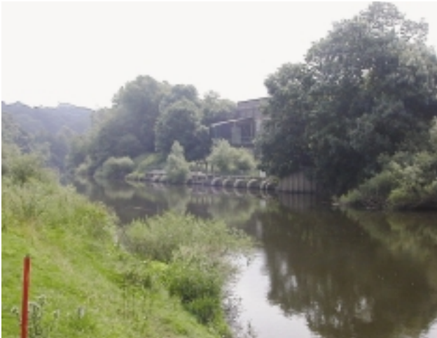
D4a Outfalls and intakes - this is a major water abstraction point (intake) occupying >25m bank-length.
