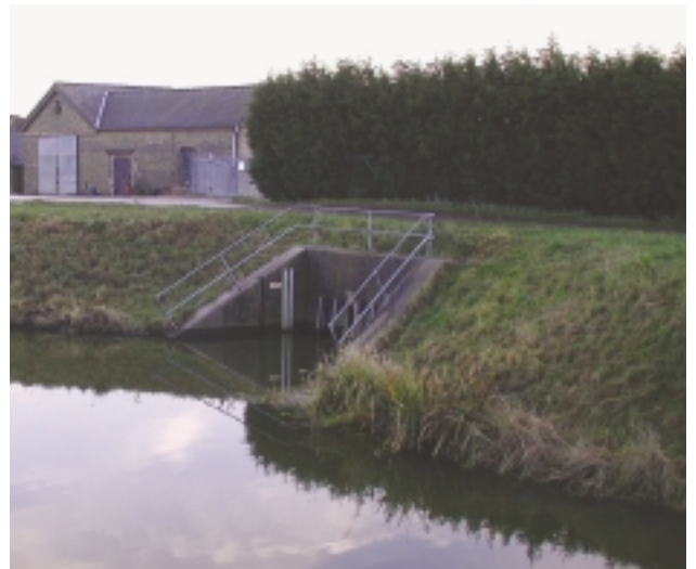
D4b An intermediate outfall, 10-25m long.
