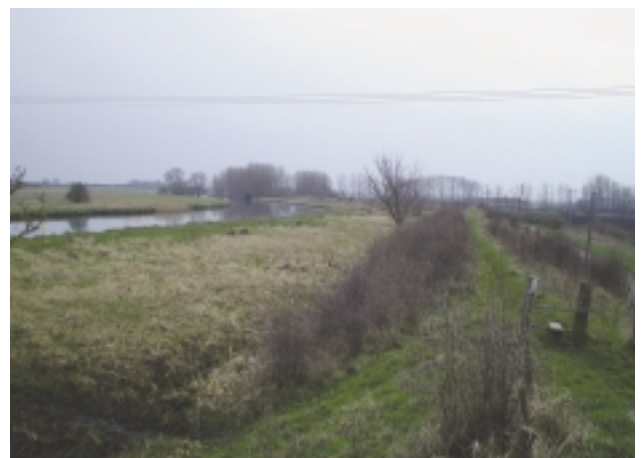
I7a Set back embankment made of earth (on right).
