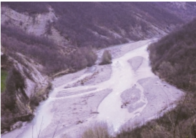
M1c Braided channel – aerial view of a highly mobile channel with floodplain absent.
