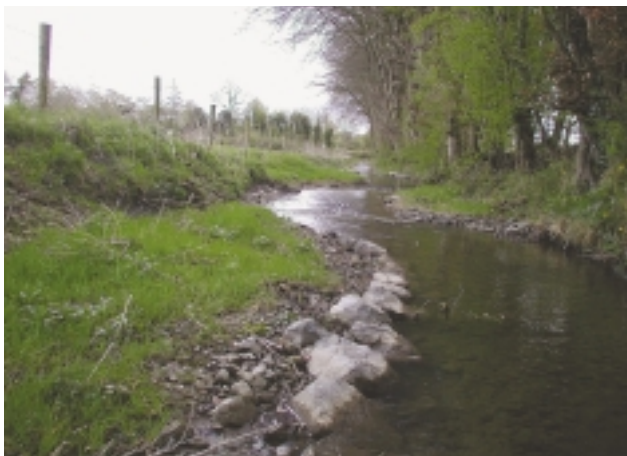
E2Cc Artificial Berm – formed by infilling an over-widened channel (here on both sides) to form a distinct two-stage (slightly meandering) channel. Note in Section P, as part of river rehabilitation works.
