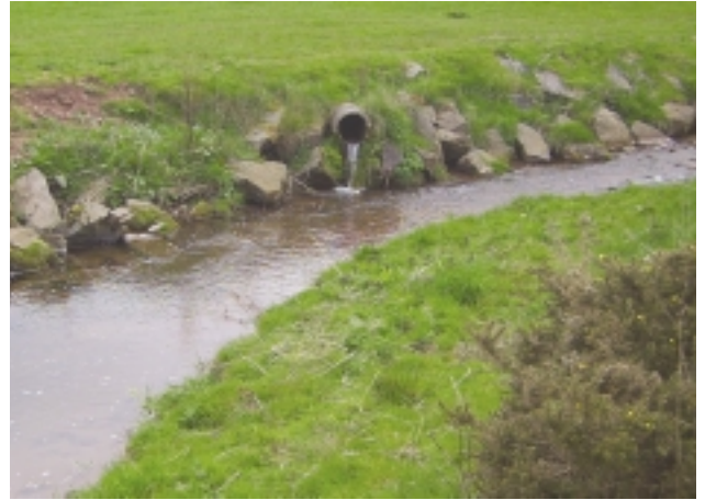
E1Md Rip-rap bank material; laid boulders with earth between. See also I6a.
