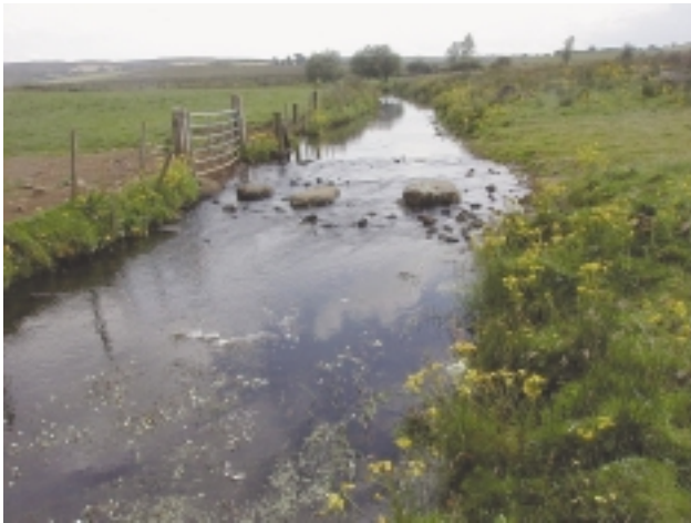
D5d Minor ford - farm track where bed and banks are of natural material, and there is no ponding from the ford.
