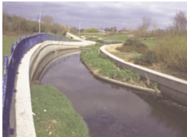
E2Cb Artificial Berm – formed by infilling wide, totally artificial, channel (here on both sides) to form a two-stage channel.
