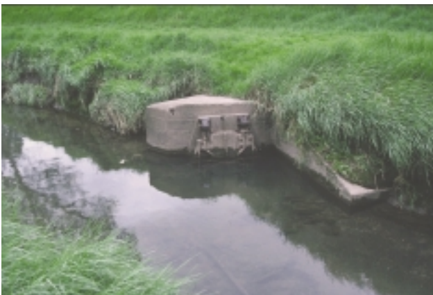
D4c Minor outfall – example of a flap-valve on a drainage channel – all such structures occupying <10m bank-length are recorded as ‘minor’.
