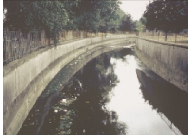
E1Ha Concrete bank material. See also A1c, E2Cb, E7Cc.
