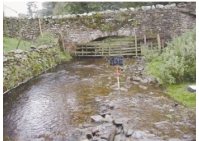
E1Lc Brick/laid stone bank material – example of stone wall bank material used in rural areas such as the Lake District.
