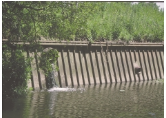
E1Ia Sheet piling bank material.
