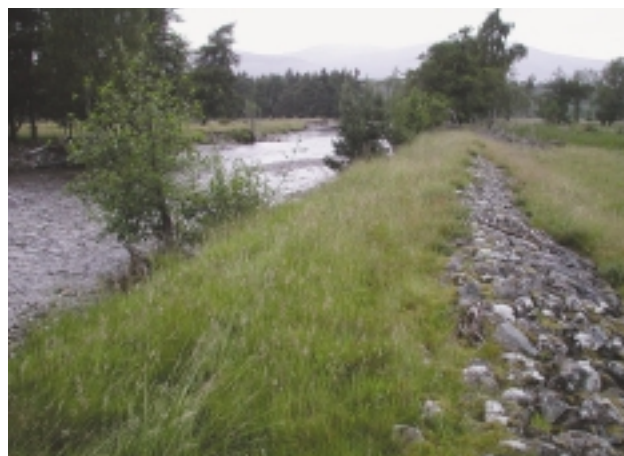
E2Db Embanked - note the rock embankment is placed on top of the natural bank. Top of embankment represents 'banktop'.
