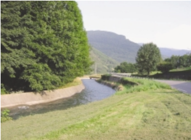
A1c Concrete channel replacing part of natural watercourse; site is obviously hugely modified but is still part of a river.
