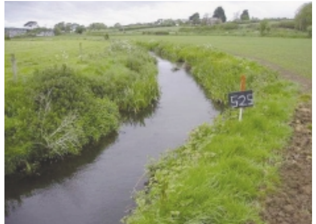
A1d Deepened and resectioned channel; site is hugely modified, but is still obviously part of a river. See also D7a.
