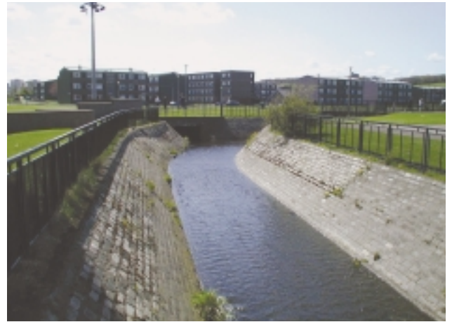
E1La Brick/laid stone bank material – cemented.
