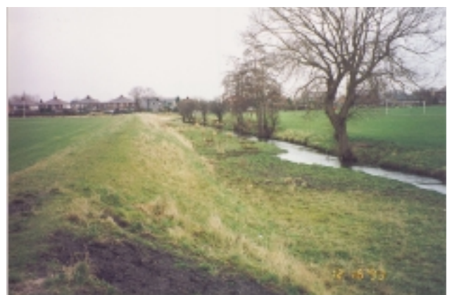
F18b Parkland & gardens land-use – includes sports fields. Note river has artificial berm and floodbank on left. Regularly spaced trees on right.
