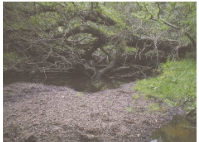
M7b Debris dam – woody debris is creating an obstacle to flow, downstream of which is a large discrete gravel deposit formed from scouring a hole below the debris dam.
