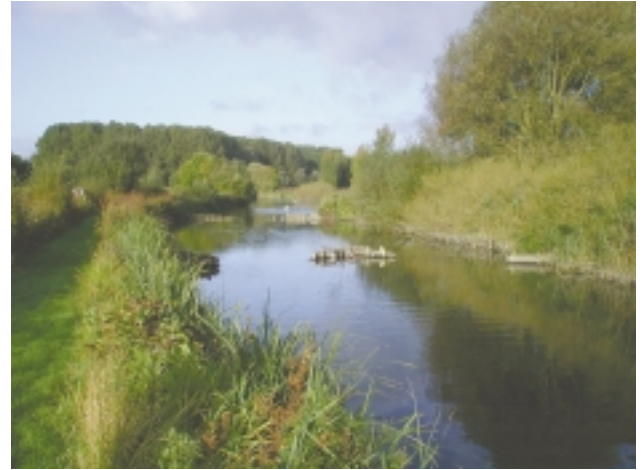
D6d Intermediate deflector/groyne/croy – example of bank, and in-channel, deflectors extending across 10-20% of the channel.
