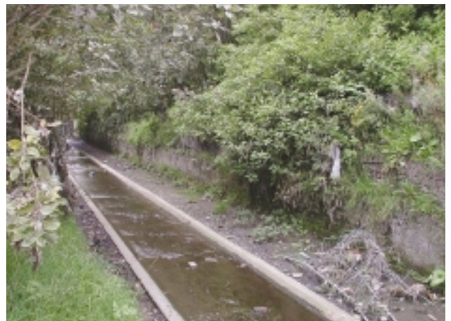
E4Jb Artificial channel substrate – concrete bed.
