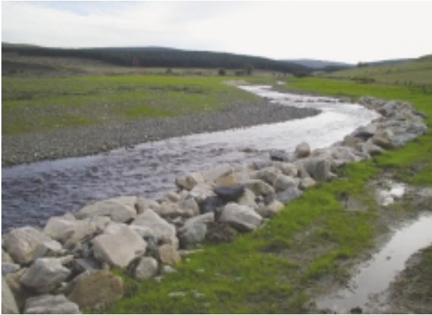
E1Mc Rip-rap bank material; tipped boulders.
