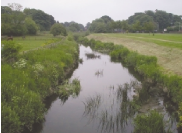
E2Aa Resectioned (reprofiled) bank – tell-tale smooth (trapezoidal) slope even though undertaken many years ago; river also over-deepened, with tell-tale ‘step’ in the profile where bed material at the base of the bank removed. See also A1a, D8a,b,c, E3Da, I6b.
