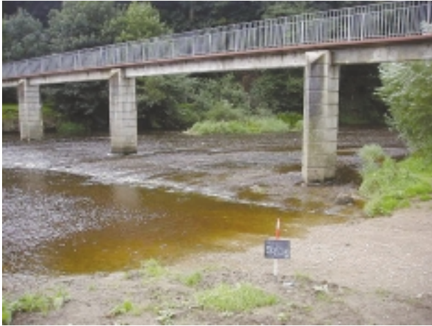
D5b Intermediate ford – note the bed is composed of artificial material, but the banks are ‘natural’ gravel. Note major bridge downstream with in-channel supports.
