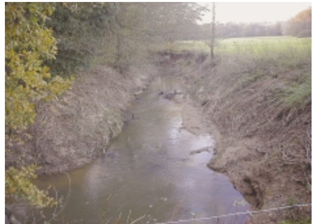
D8b Over-deepened channel – obvious signs include the slumping of the artificially steep banks and the channel width/bank depth ratio is <4:1 .
