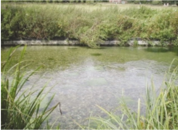
E1Oa Fabric bank material – non-degradable sheet ('nicospan'). Note tall herb bank vegetation above, so record structure as 'simple'.
