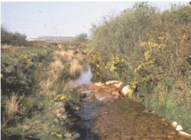
D1c Major weir/sluice – despite small size, the weir structure is 'fixed,' and does not leak water. Note scrub and short grass on right, and short grass and tussocky tall grass on left – both with simple bank vegetation structure. Water upstream is impounded.
