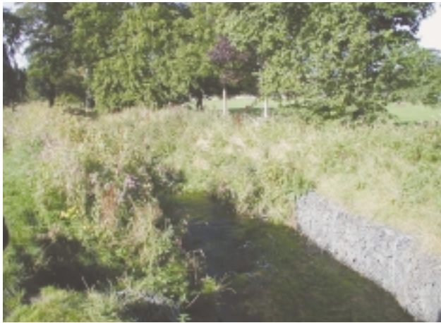
E1Ka Gabion bank material – boulders/cobbles in wire baskets. Typical example of use in protection of the bottom half of a bank.
