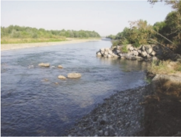
D6c Intermediate deflector/groyne/croy – an example of a boulder deflector extending across 10-20% of the channel.
