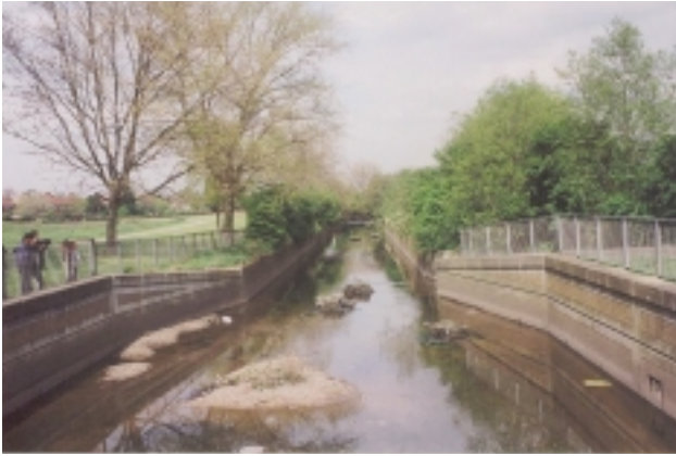
E7Cc Unvegetated mid-channel bar – example in urban stream. Note concrete bank material and presence of shopping trolleys (urban debris; but not predominant).
