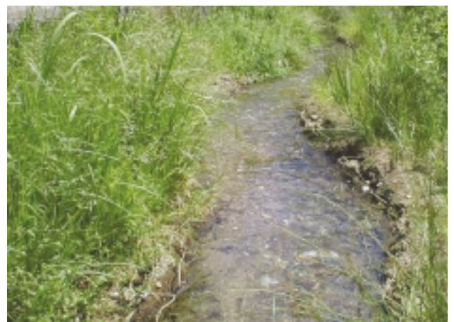
E1Pe Bio-engineering bank materials – here bio-degradable hessian has been used in combination with reed planting and other vegetation.
