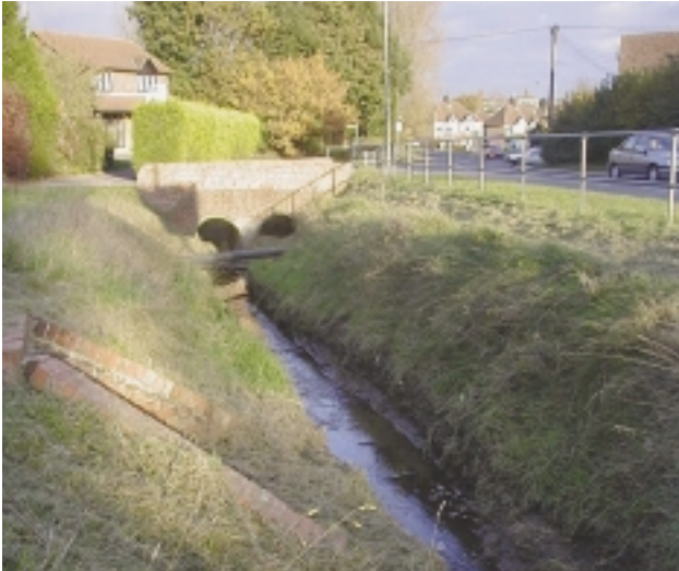
F15a Suburban/urban development land-use - rivers surrounded by houses or industrial buildings. Note minor outfall and resectioned bed and banks.
