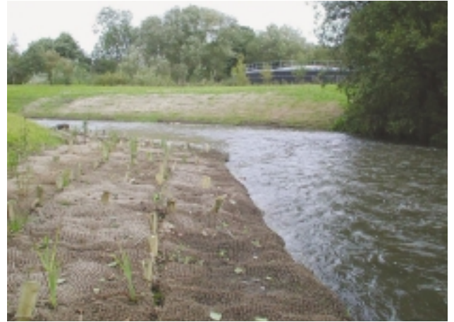
E1Pa Bio-engineering bank materials – bio-degradable matting with vegetation planting. Record bank vegetation structure as 'bare'.
