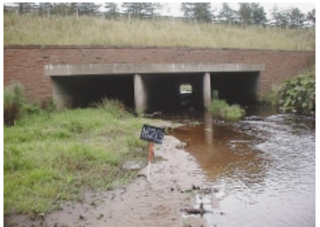
K2c Unvegetated silt deposit – surface has >50% vegetated cover, but the underwater part of the deposit has no vegetation.
