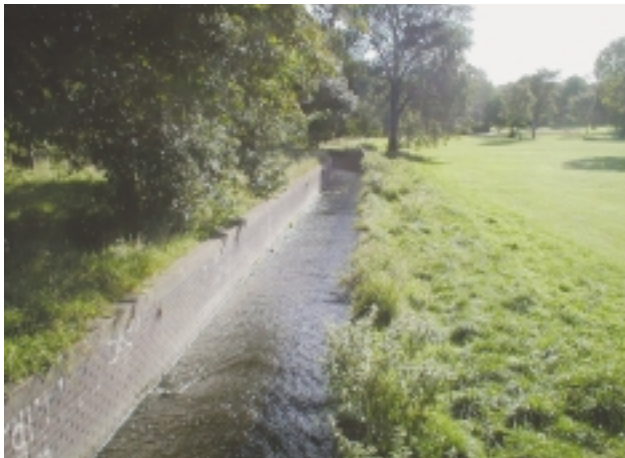
E1Lb Brick/laid stone bank material – cemented bricks. Note parkland land-use on right.
